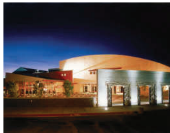
A uniform lighting approach creates visual interest and assists with wayfinding.
