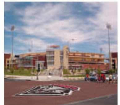
Major intersections could become more pedestrian and visitor friendly by adding color and logos to create interest and identity.
