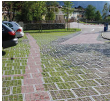
Porous paving is a good option in parking lots to help reduce the stormwater runoff.
